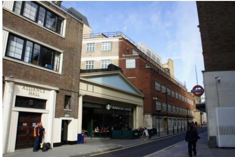
Fig.2: A single storey building erected over a former open section of sub-surface railway, in Palmer Street, Westminster, London. Such a scenario as this can be representative of other locations on a metro system or other systems. Source: Nathan Darroch.
