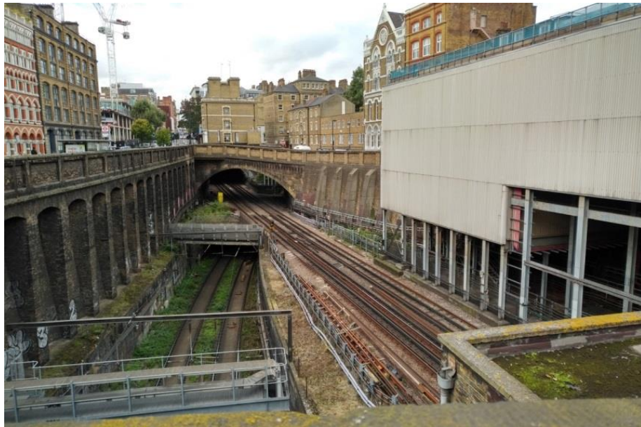
Fig.8: Photograph, looking north, showing Ray Street highway bridge (centre distance); LU Metropolitan Line railway (to the right); and Network Rail Thameslink railway (to the left).
