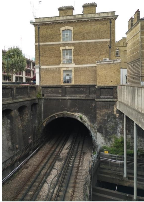
Fig.12 photograph showing 54 Farringdon Road, located over the sub-surface Metropolitan line tunnel, which on approaching the tunnel is in an open cutting. To the bottom right, below the Metropolitan line is the Network Rail Thameslink route.
