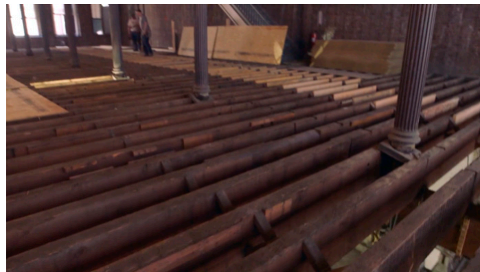
Figure 3. Historic joist floor.
