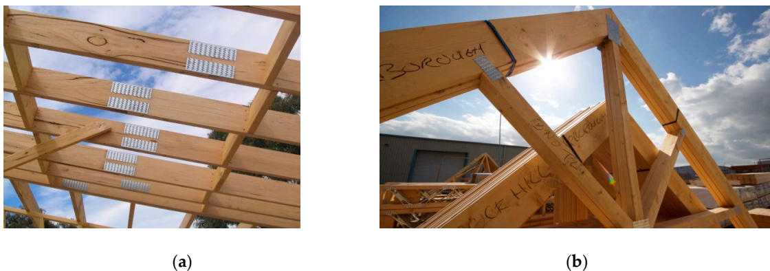
Figure 16. Examples of connections made with nail-plates [51,52].
