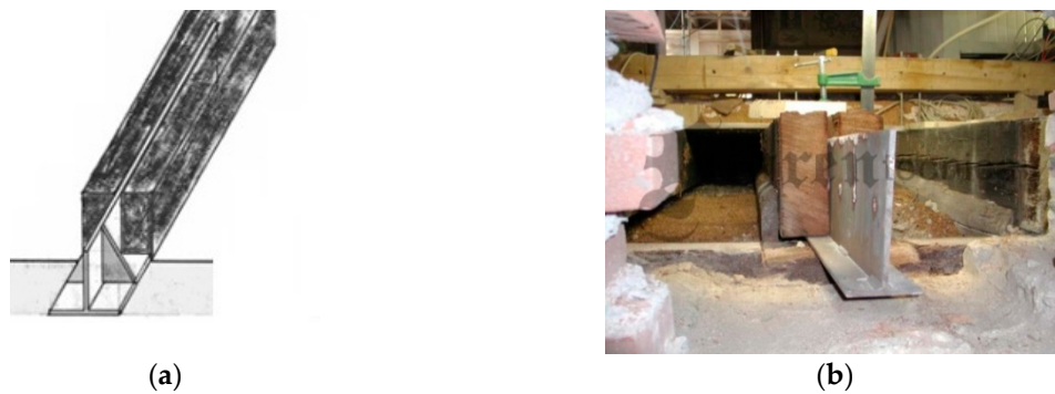
Figure 12. A stainless steel flitch plate inserted into a timber beam and bolted side-to-side: detail of the steel profile used at the beam ends [44,45].
