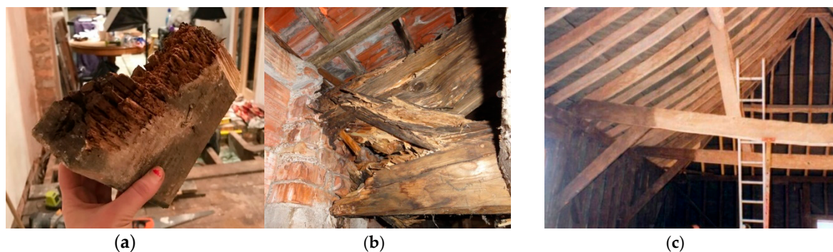
Figure 6. Examples of damage in timber structures: (a) and (b) Rotting wood at the beam-ends, and at the joists in timber roof truss; (c) Deformed timber tie in a frame of a roof structure because of over-loading.
