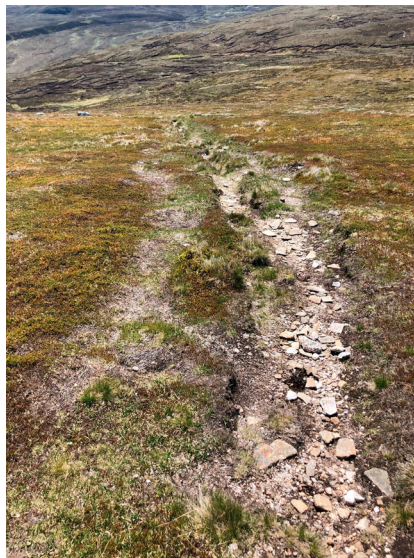
Figure 2. As the main path (right) has become an unpleasant walking surface, walkers go 'off-path' creating a new track (left).
