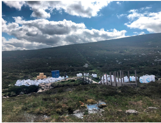
Figure 5. Bags of stone and a new bridge deposited on the hill by helicopter. This illustrates the logistics and cost involved in upland path management.
