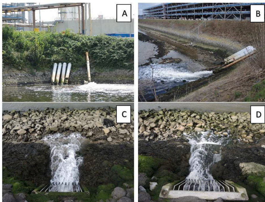
Fig. 1. Brine discharge points (A & B: IEX and RO effluents from DWP Botlek, C: IEX effluent from DWP Maasvlakte, D: RO effluent from DWP Maasvlakte).
