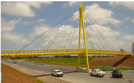
Figure 1. Full scale cable stayed bridge.
