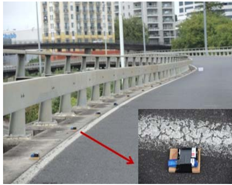
Figure 6. MEMS tri-axial accelerometers on the bridge deck (inset: accelerometer/D-cell battery unit).
